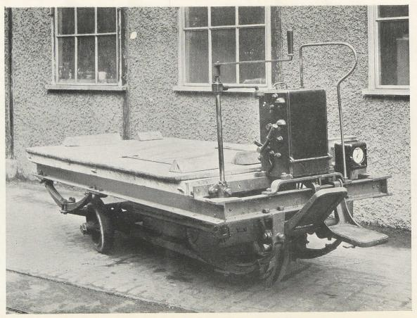
A THREE-WHEELED TYPE OF ELECTRIC TRUCK
