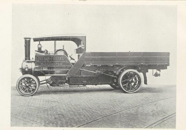
A 5-TON WAGON WITH OVER-TYPE ENGINE.
