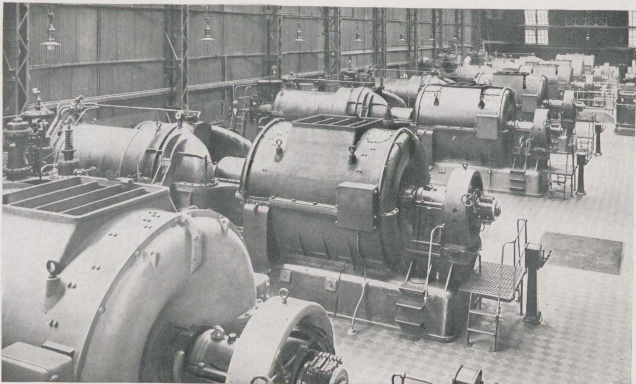
Fig. 181.—Inside a Power Station: The Carville Power Station, showing Parsons Turbo-Alternator sets
