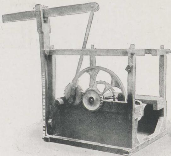
Fig. 19.—Model of Watt's Sun and Planet Motion
