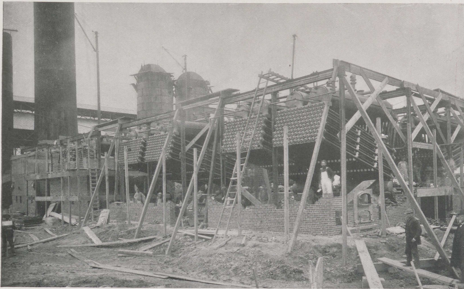
Babcock & Wilcox Boilers at Pennsylvania Steel Co.'s Works, Sparrows Point, Md. 4,000 H. P. in Process of erection, 1888.
