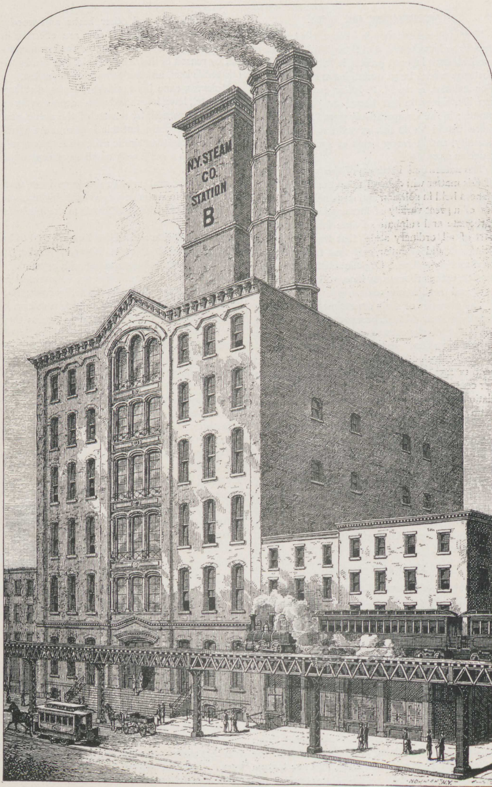
New York Steam Company's Station B, completed. Containing 16000 H. P. of Babcock & Wilcox Boilers.
