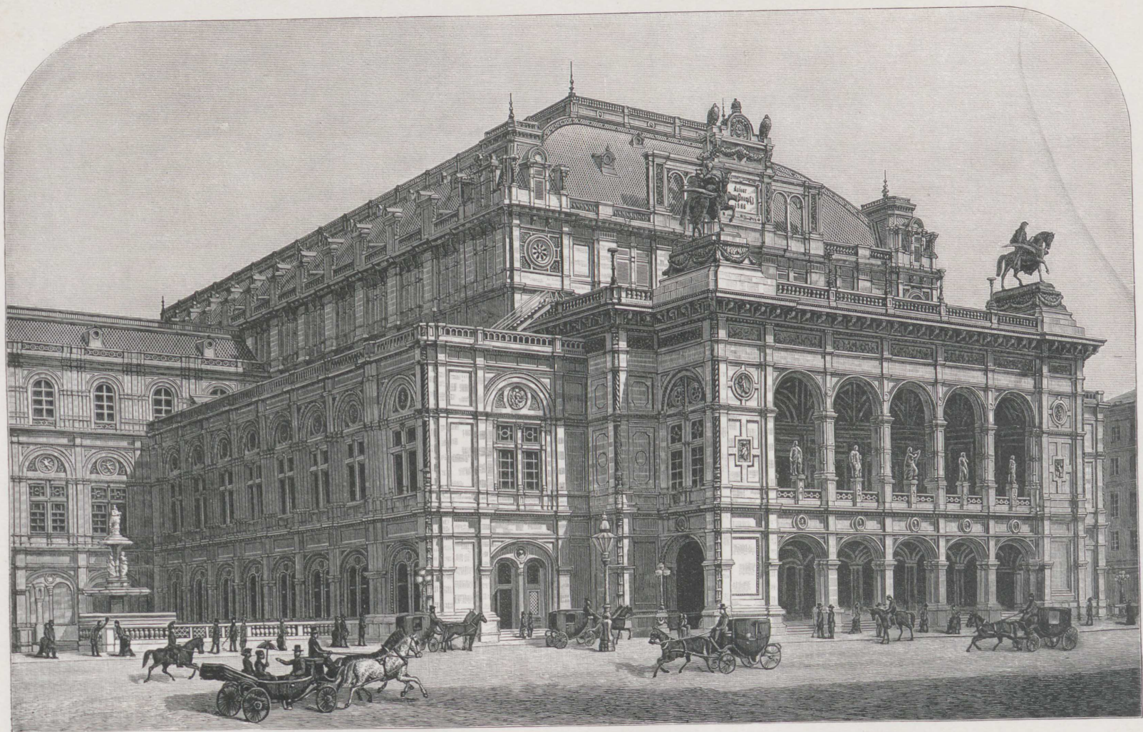
Vienna Opera House, Vienna, Austria, lighted by electricity. Power furnished by 1192 H. P. Babcock & Wilcox Boilers.
