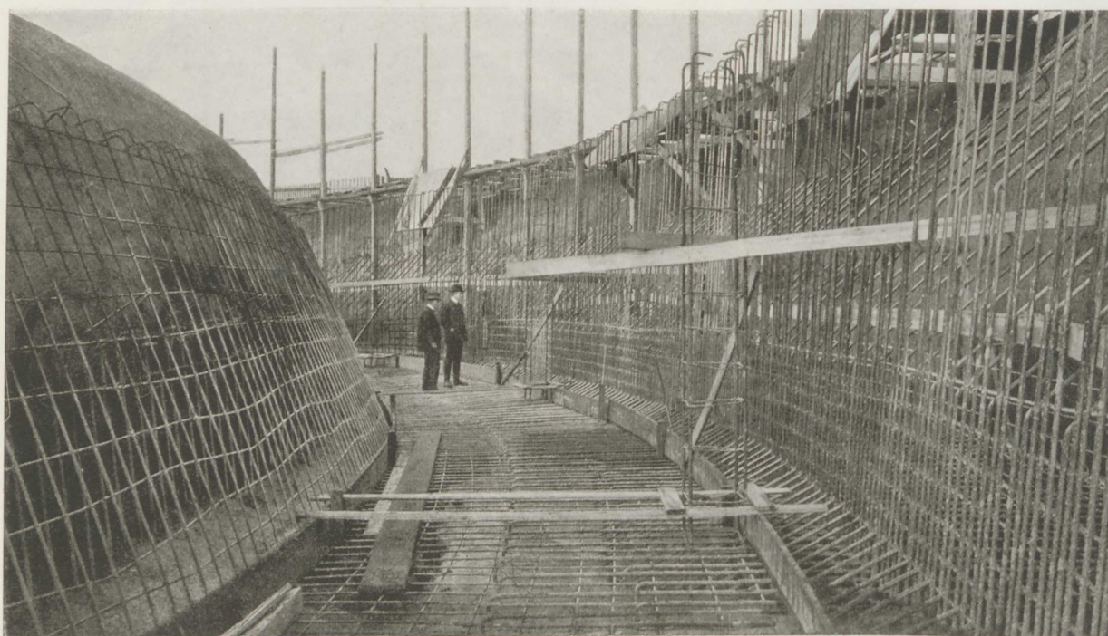
RINGBASSIN FOR GASBEHOLDEREN I FUHLSBÜTTEL. Diameter 60 Meter.
